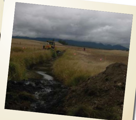
Stream Restoration - Hoyt Creek (Photo by Ryan Aashiem)
